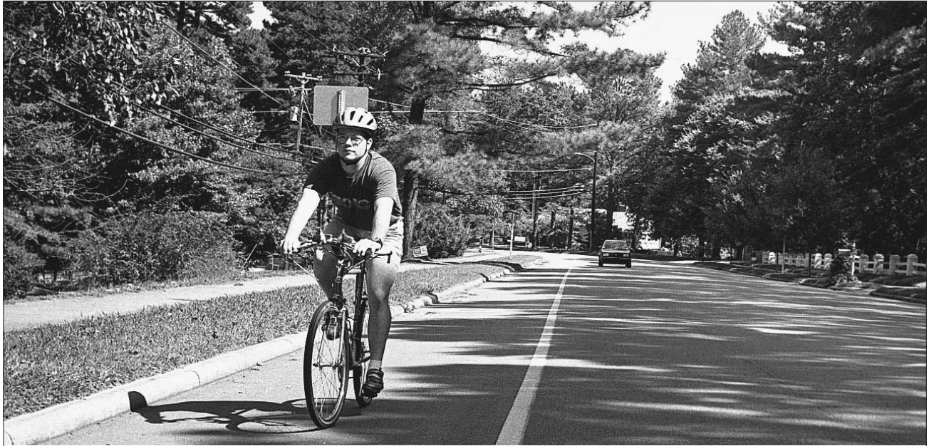
Bicycle lanes are portions of the roadway designated exclusively or primarily for bicycles.
