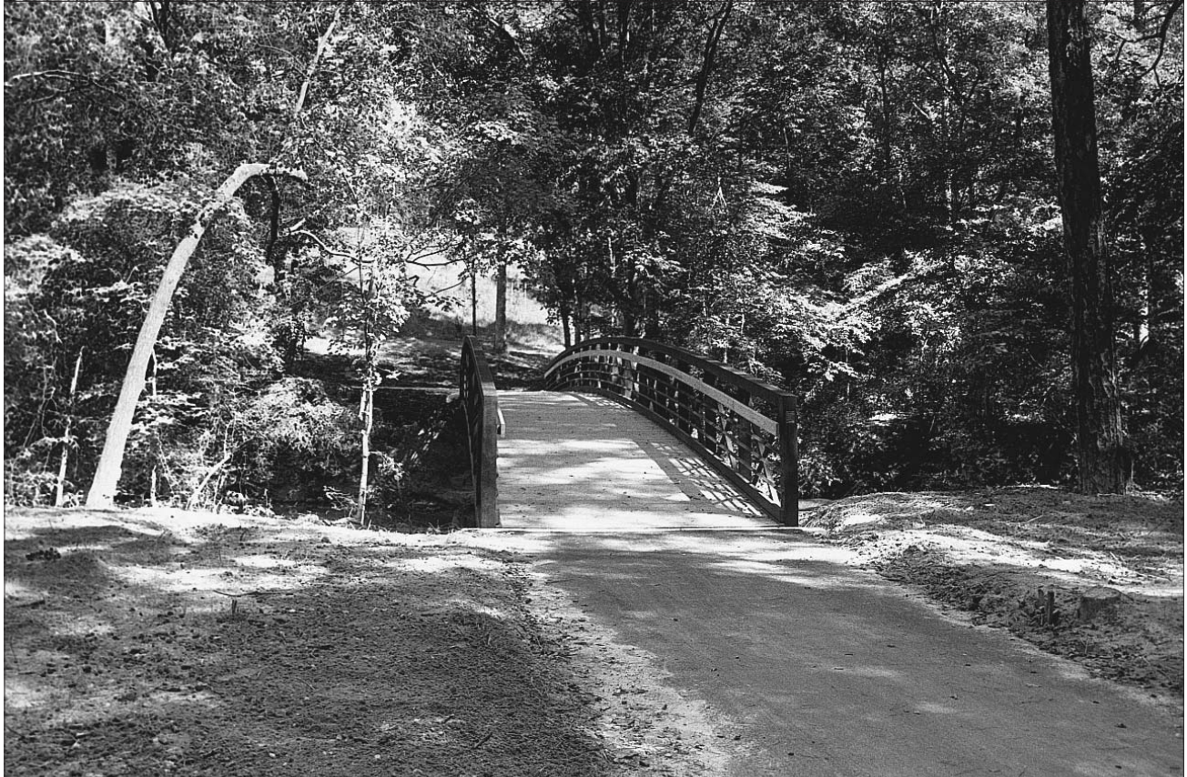
An example of a bicycle-pedestrian bridge.
